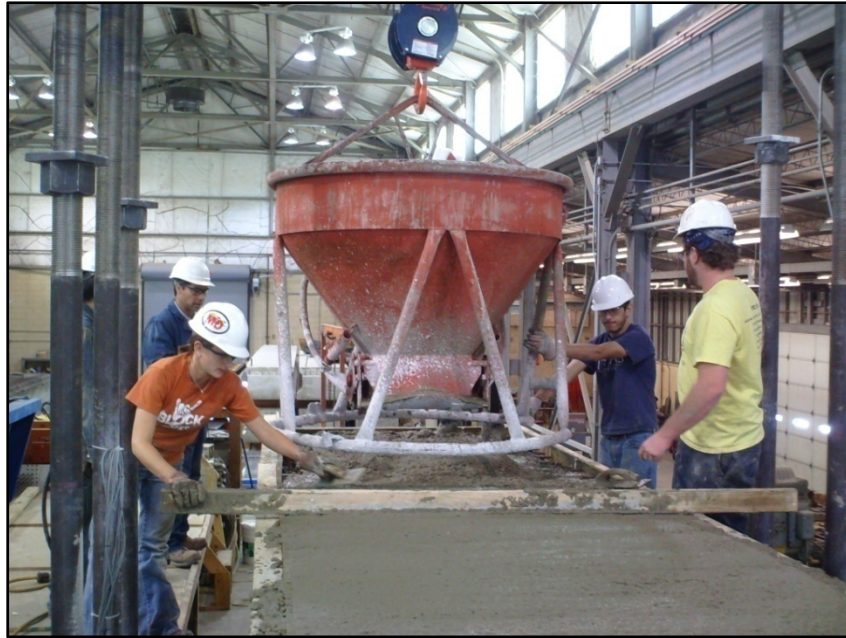
Figure 3-11 Casting of beam RF-3R-9(c).
