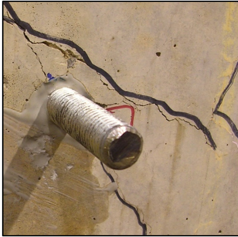
Figure 3-21 Threaded rod epoxied into predrilled hole in trapezoidal box beam.
